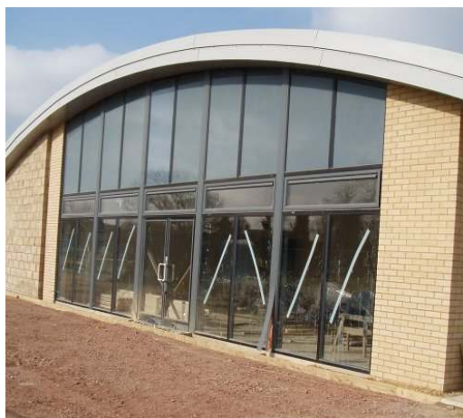
The front of the new Pavilion
